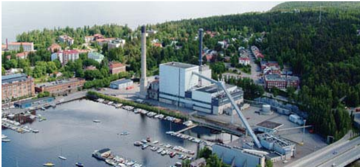
Power Plant Naistenlahti 2 (Tampere, Finland)
